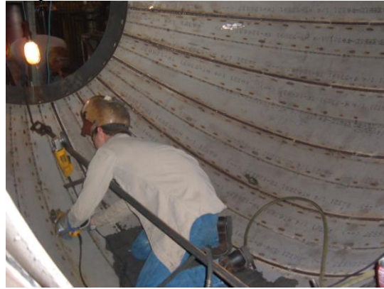
Shop Fabrication of Shroud Bottom Section
