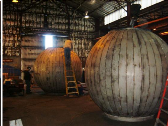
Shop Fabrication of Shroud Bottom Section
