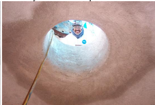
Refractory Installation Top Inlet Nozzle
